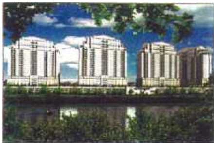
Millennium, O'Neill Properties mixed-use development along the Schuylkill River in Conshohocken, Pa., will feature more than 1,000 residential units, 200,000 square feet of office space and light retail.
